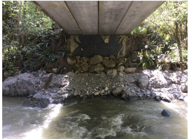
Right Bank Abutment when facing downstream
