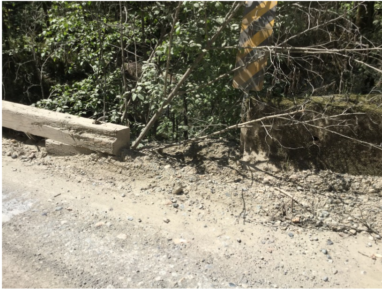
Upstream left bank barrier alignment
