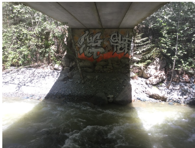
Left Bank Abutment when facing downstream
